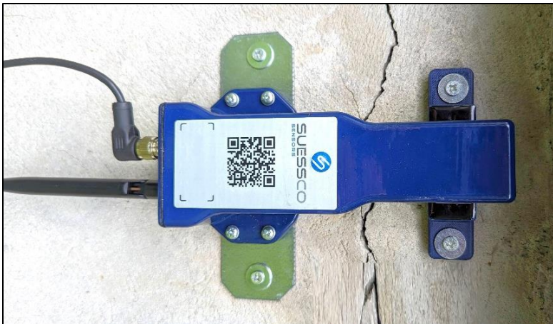
Reference crack application
